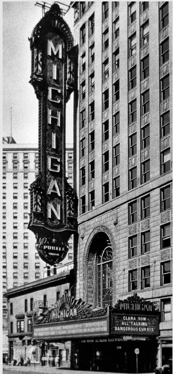
The magnificent Michigan Theatre in Detroit before it was turned into an unlikely parking garage decades later.
